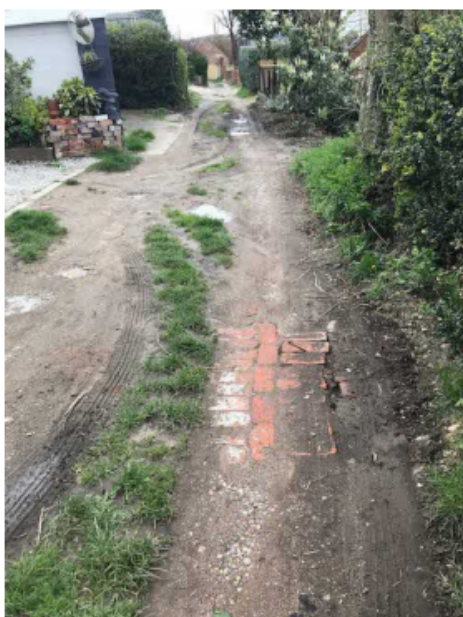
Fig. 18 Poor condition of Victoria Passage with ad hoc repairs – bricks used to stabilise fragile passage surface.
